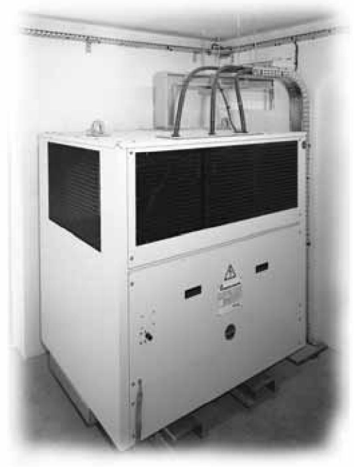
figure 4 - LV connections with PBT on enclosure
